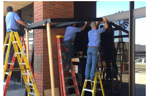
Building Maintenance installing an awning at City Hall.
