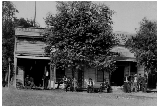
When Roger Dunham is not managing capital projects, he is managing construction upgrades to his new business venture, ask him about it! (Photo Circa 1890)
