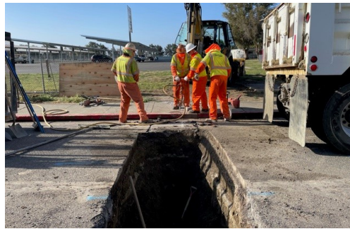
Water Distribution team installing a new fire hydrant.
