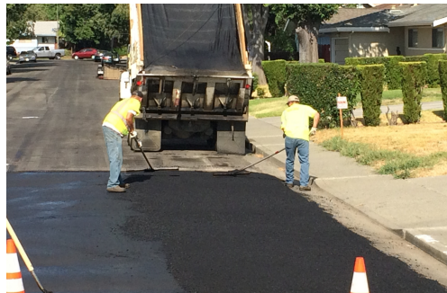
Streets team making a permanent street repair after water maintenance.
