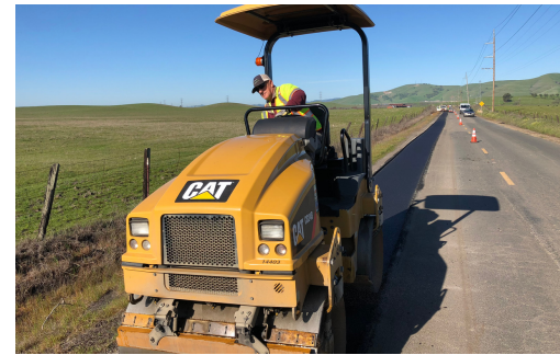
Pete Brooks compacting asphalt.
