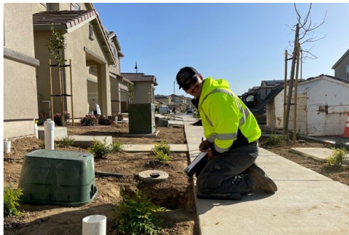
Jarred Allen installing a new water meter.
