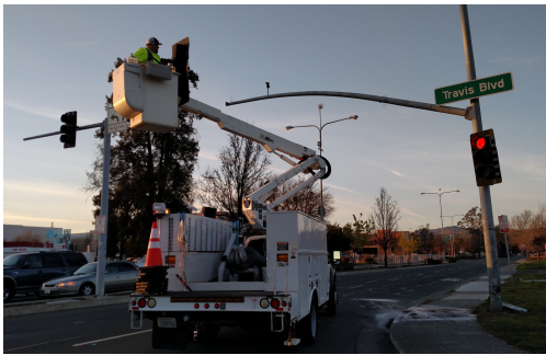
Traffic team working on a damaged traffic light.
